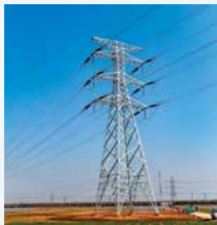
Tower and substation EPC
